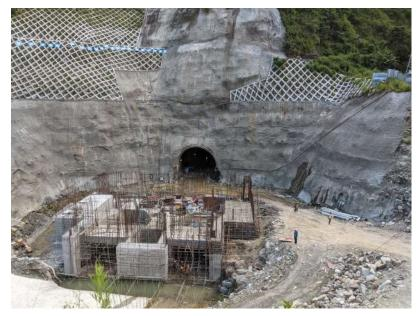
clearing and started rock bold work for permanent support.
