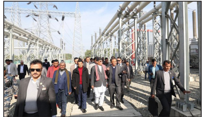
INARUWA SUBSTATION : Era of High Voltage
