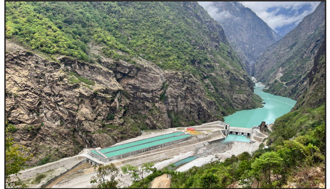
COVERSTORY: LOSS AND DAMAGE: Upper Tamakoshi A Case 22
