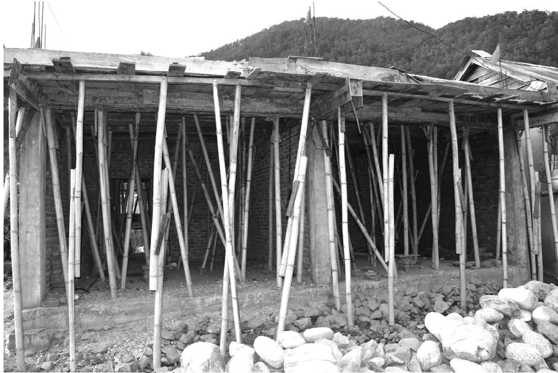
Construction in progress in Bhorletar
