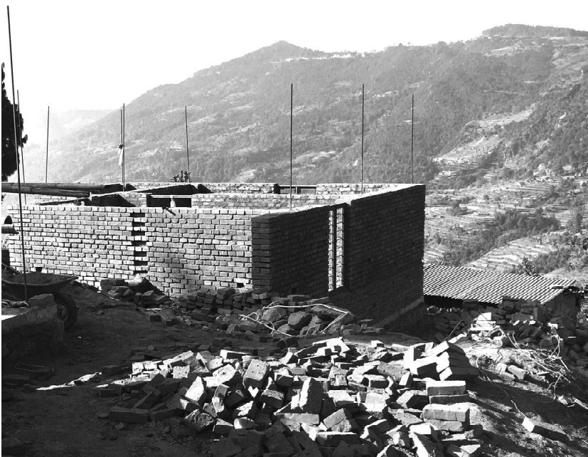
Reconstruction in progress
