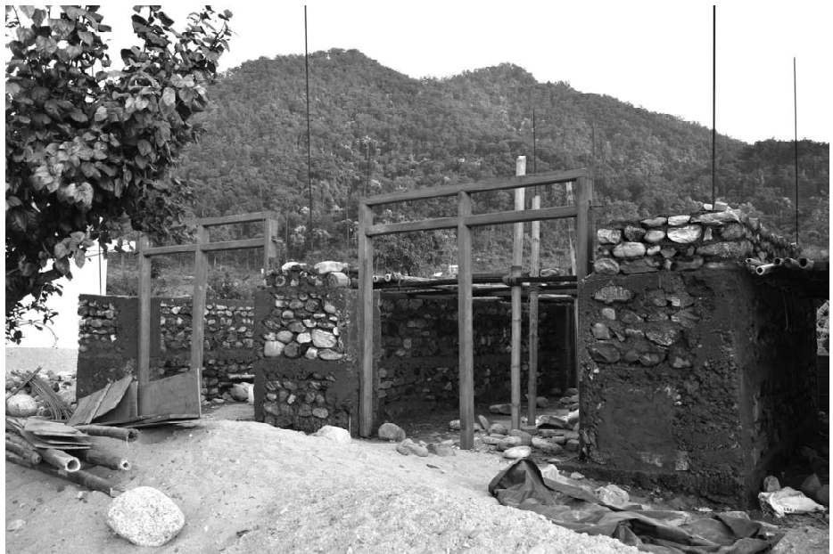
A house under construction
