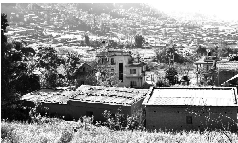
Waiting for reconstruction
