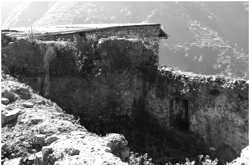
Debris of house
