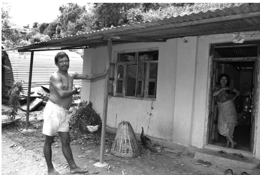
A new house of Thula Kanchha Sarki constructed with government grant
