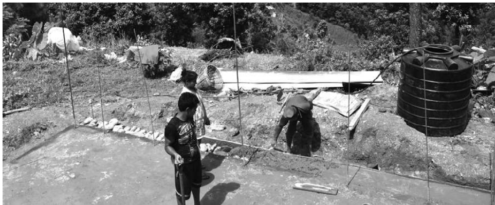
Laying the foundation
